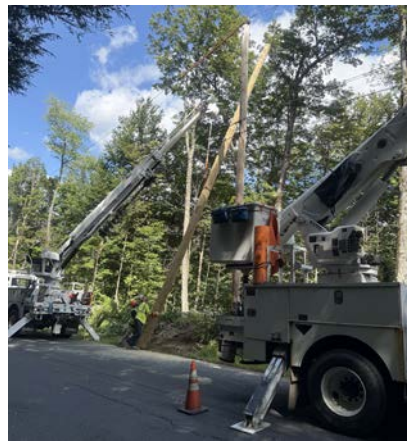
A new pole is hoisted into place on Town Hill Road.
