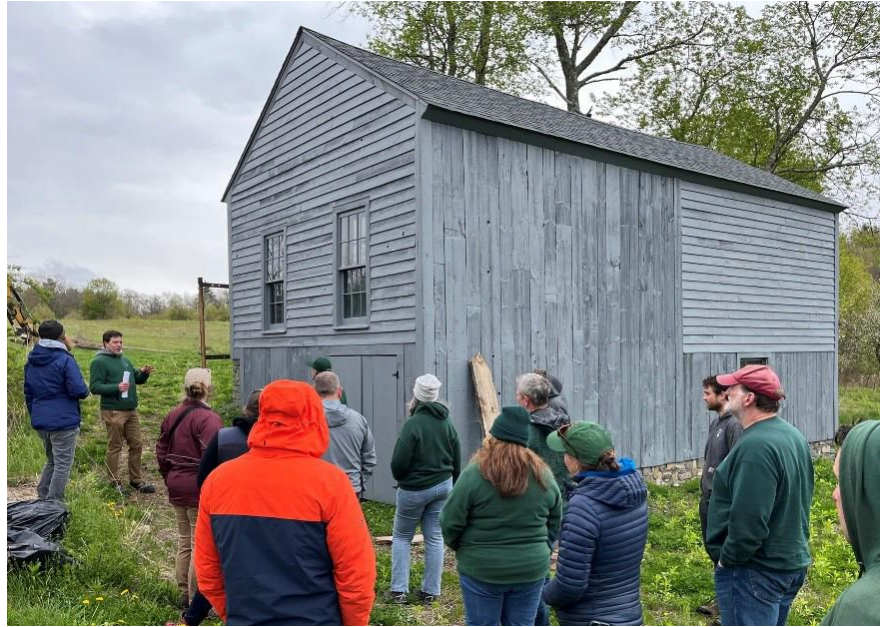
Kevin Allen revealing the newly-restored exterior of the abattoir.
