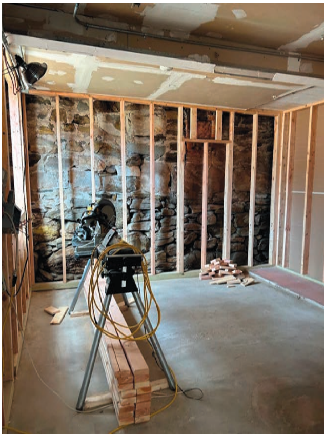
The future kitchen, formerly the oil tank room
