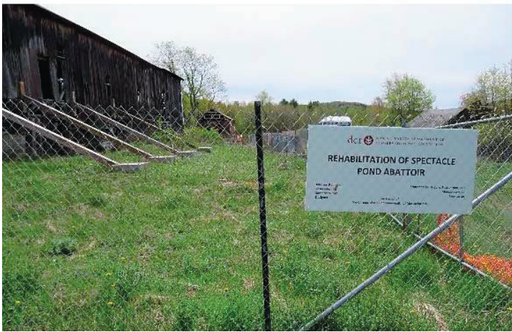
The building is fenced during restoration
