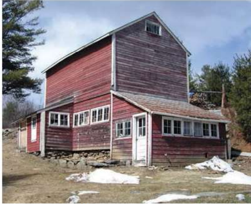
The old Porter & Carter shop, still standing. Photo Sandisfield Then & Now, 2011
