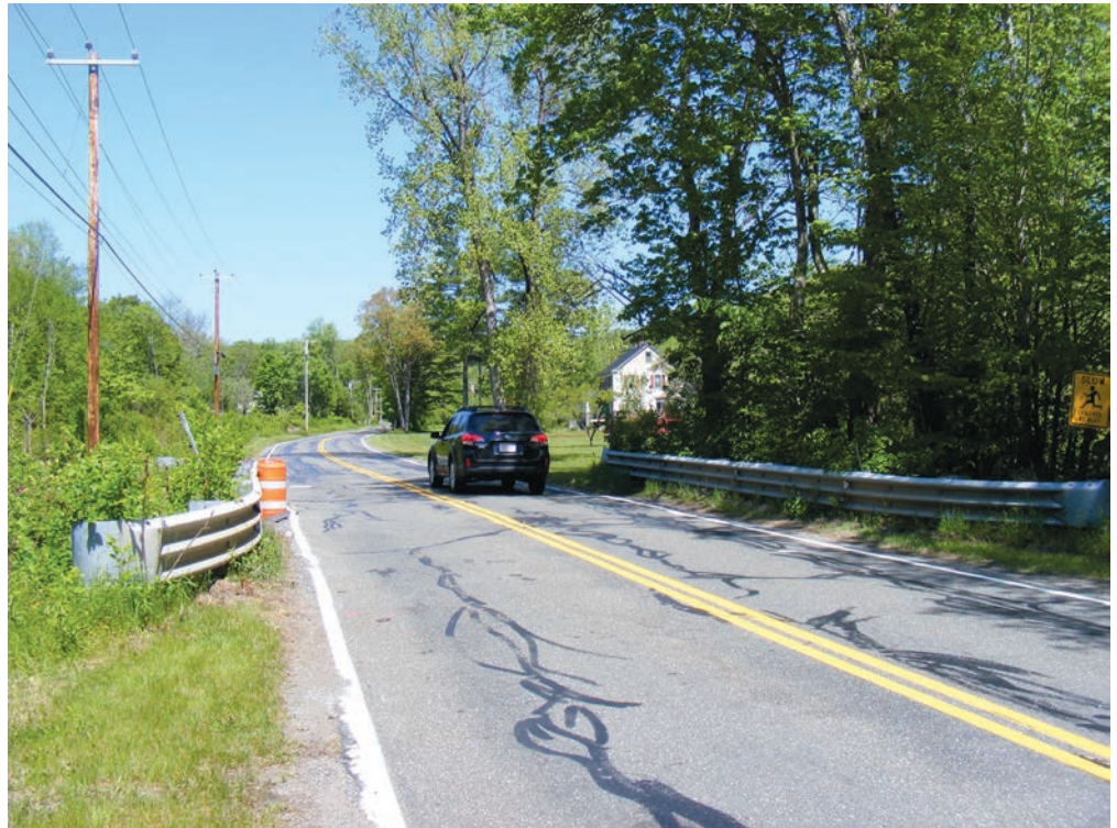
The site of the culvert repair.
