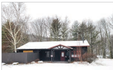
The former MJ Tuckers, which will be demolished.
