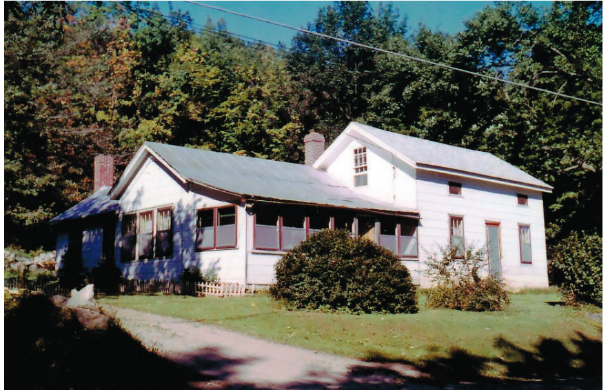
The former New Boston Congregational church parsonage on No. Main St./Route 8, as it appeared in 1961. Rev. Whitney lived there 1919-23 and owned it for five years, selling in May 1944. The house was demolished in 2009.
