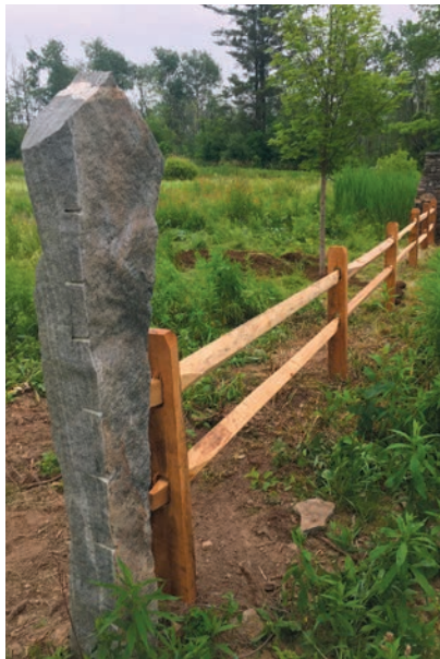
The new split-rail fence near the Park's entrance.
