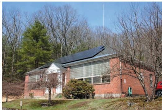
Town Hall Annex capped by its new solar panels.
