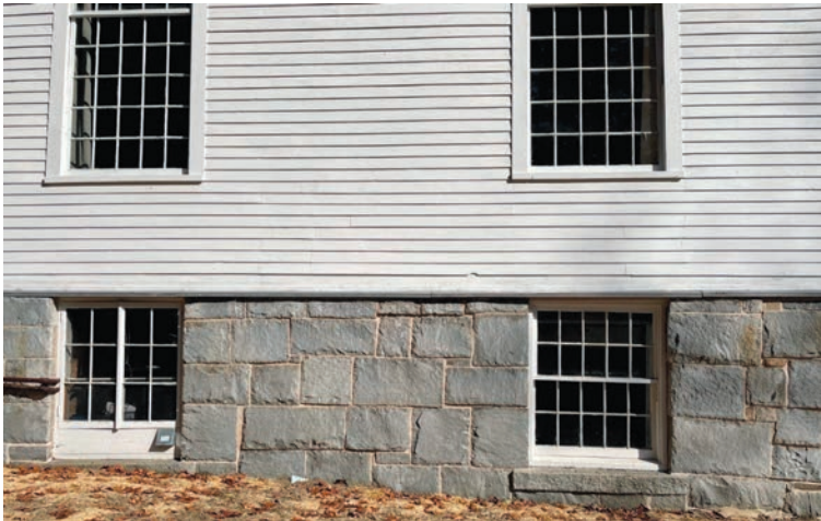
Overall repointing of one elevation of the Sandisfield Arts Center.
