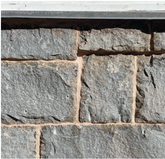
Detail of the repointing mortar
