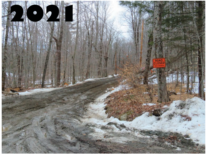
Hammertown Road at Cold Spring Road
