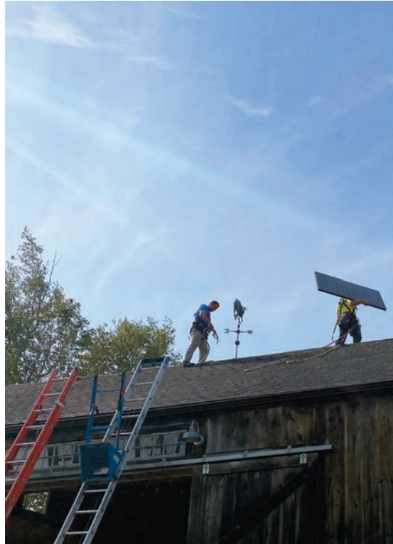
The installation begins! Photo: Simon Winchester
