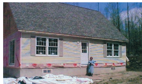
The house being assembled.
