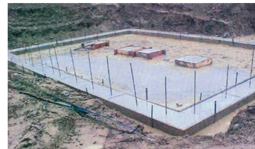
The foundation poured.
