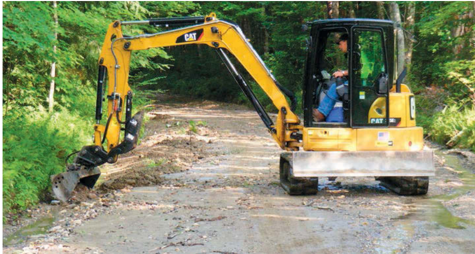
Ralph Leavenworth of the DPW carves out a deeper runoff ditch on Silverbrook Road. Photo: Bill Price
