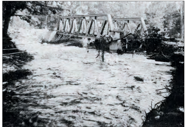
During the 1955 flood, all of the road leading to the bridge was washed away, but the bridge stood like an island.
