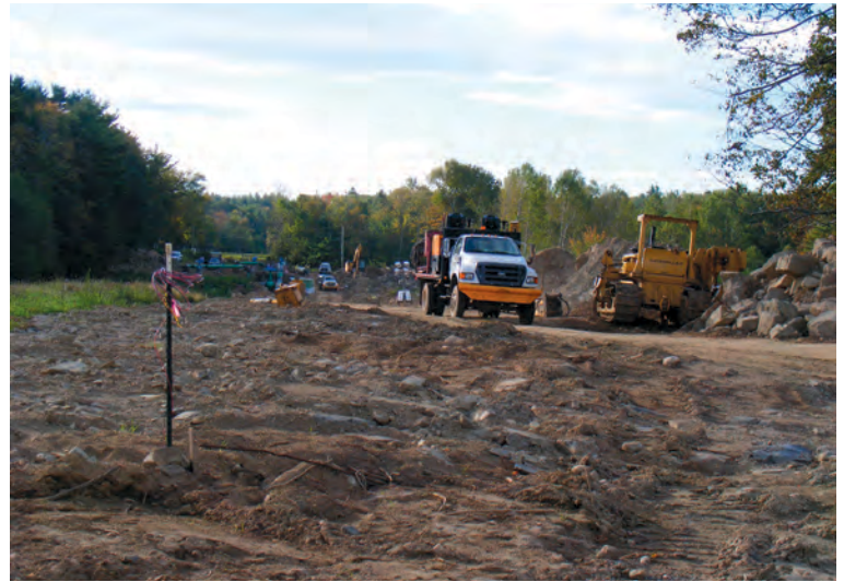
After The same place, with the pipeline underground.
