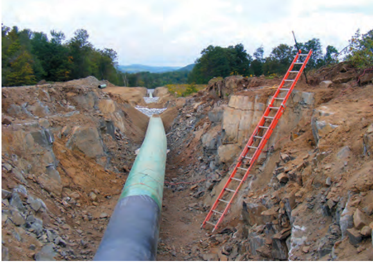
During Where the pipeline crossed South Beech Plain Road, Tennessee Gas had to blast through Sandisfield's solid granite. The ditch was about ten feet deep here.
