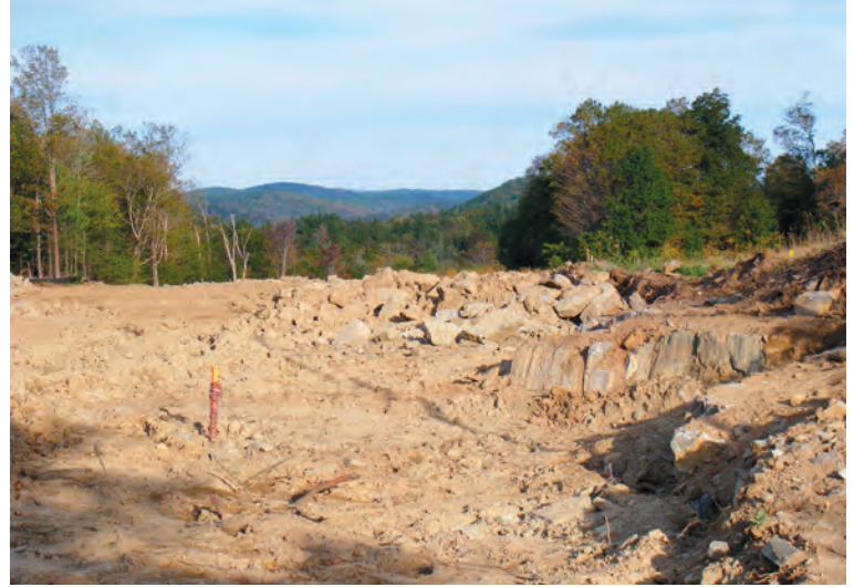
After The same place, after the ditch had been filled in and the pipeline buried. A piece of granite on the right side of the photo can be seen in the other photo with the top of the ladder leaning against it.
