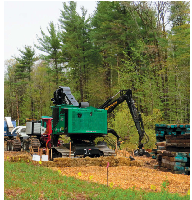
In line, clearing trees and brush.
