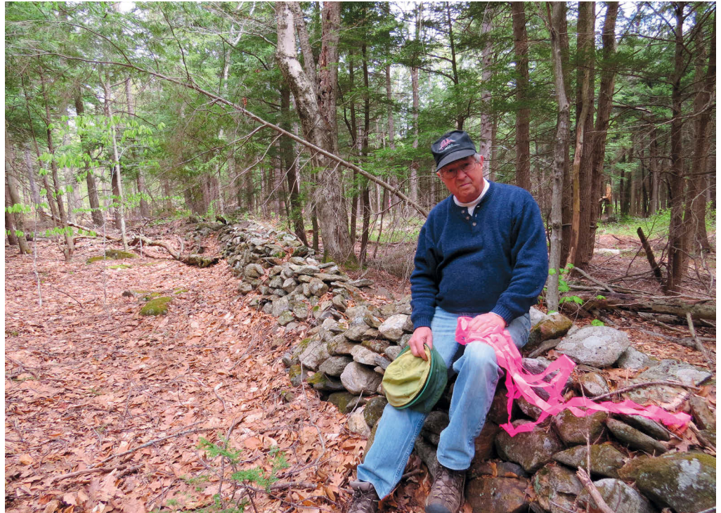
Author Ron Bernard's home on Cold Spring Road is in the middle of the construction project. This 200-year-old stone wall on his property will be demolished for a "holding space." TGP has promised to rebuild the wall, which will make it a new wall.
