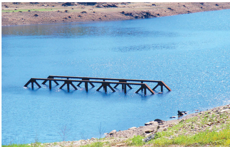
July 29. The old Rt. 8 bridge across the Farmington emerges out of the lowering Colebrook Reservoir.
