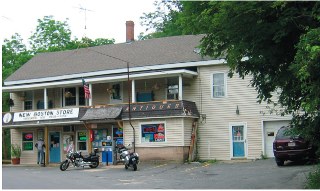
The New Boston Store, 2010, while still open for business.
