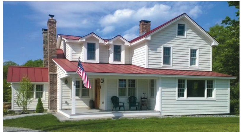
The Hubbard house as it appeared in 1985, left, and as renovated, 2015.
