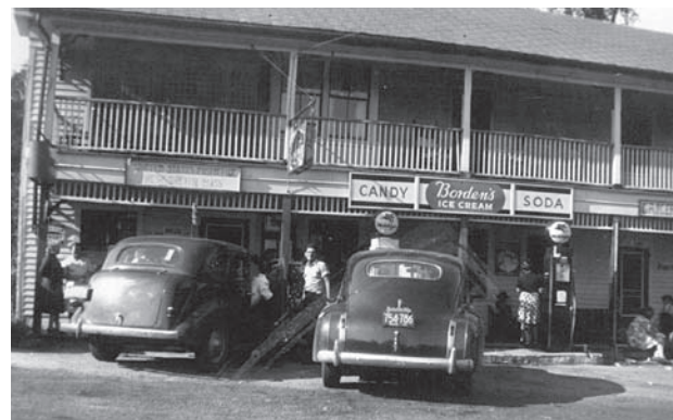
Above: The New Boston Store, about 1944
