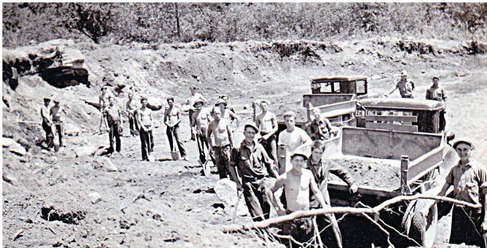
Members of the 196th load gravel for construction of the dam at York Lake, c. 1934. (David Kinne / Bernie Drew Collection)
