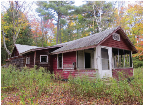
The Flint Cottage, No. 144, last October, before demolition.
