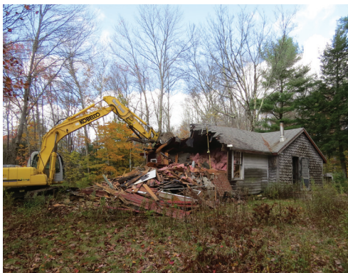
Good-bye Old Cottage. The disappearance of No. 144.
