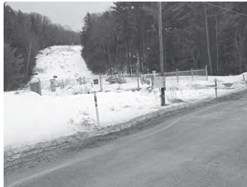
The pipeline is a 75-foot pathway through the woods with two gas lines buried a few feet underground.
