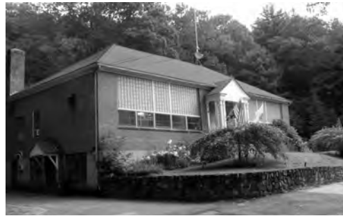
Town Hall Annex, 2013
