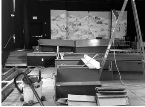
Getting down to the subfloor. Photo: Alice Boyd
