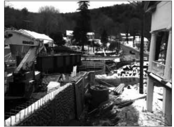
The progress of the bridge, looking east across the Farmington.
