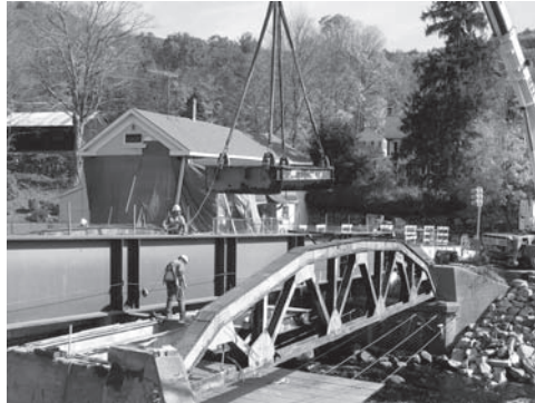
One section of the truss is removed.
