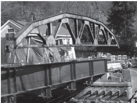
Still lifting the side rail.
