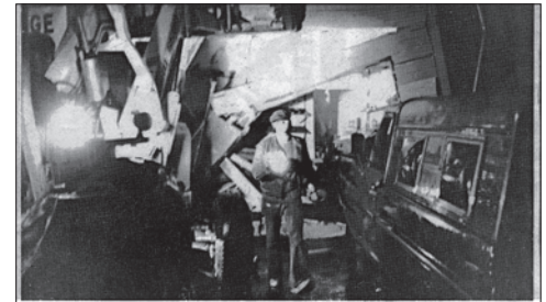
Store Front Demolished
