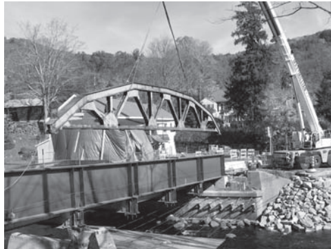
Lifting the green side rail up and over.
