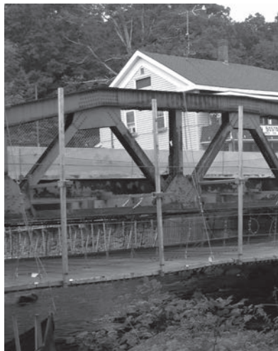
Bridge as it is.
