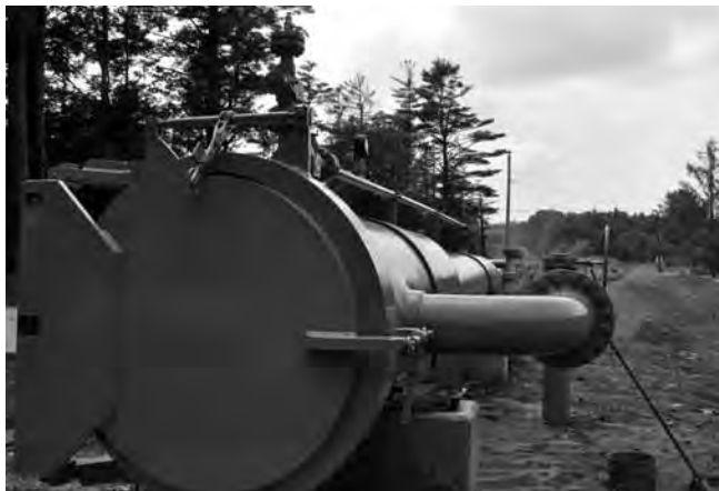
Geopig enters tube here...
