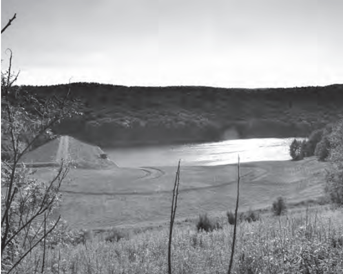
Clam Dam on Hammertown Road
